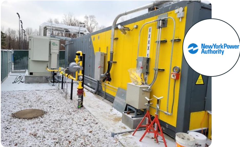
Thermal Storage Based Co-Generation Hybrid charging: Exhaust gas and electricity
